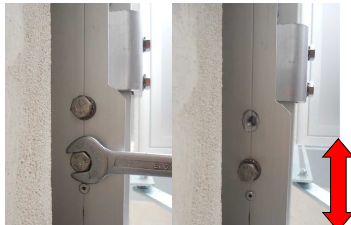
Fig. 2: Configuration of fastening screw union of the TAM2 door case
