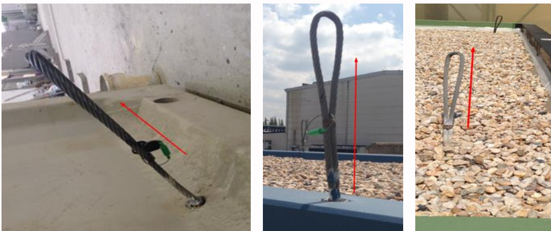
Fig. 24 Examples of permissible pull direction
