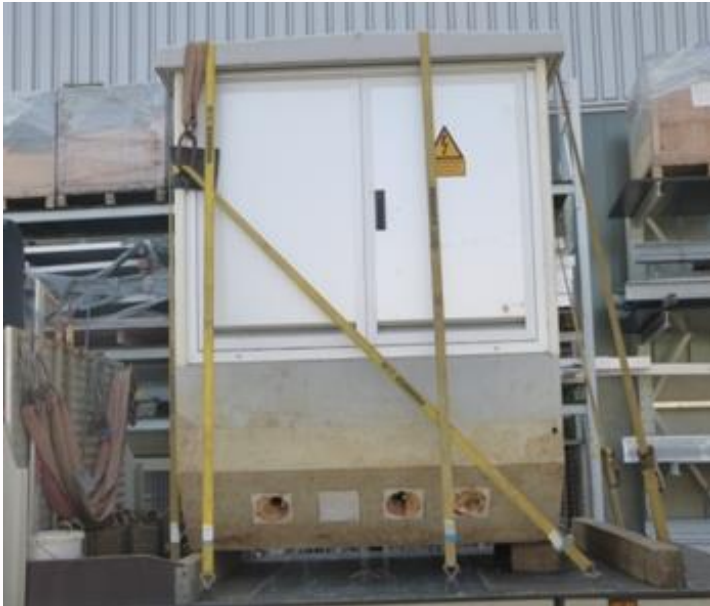
Fig. 12: Friction slinging (left) and passing the lifting accessories through (on the right)
