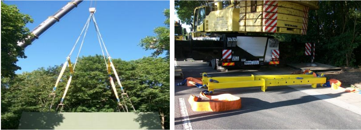
Fig. 30 Spreader beams
