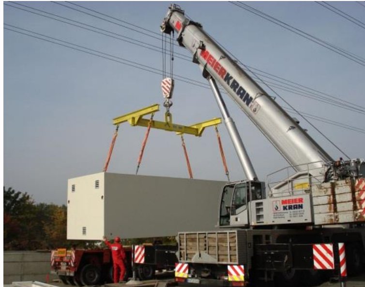
Fig. 28 Supporting beam (H-beam)
