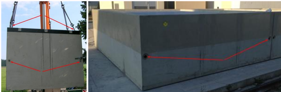
Fig. 7: Lifting inserts for lifting and securing the loads separately (left) and combined (right)
