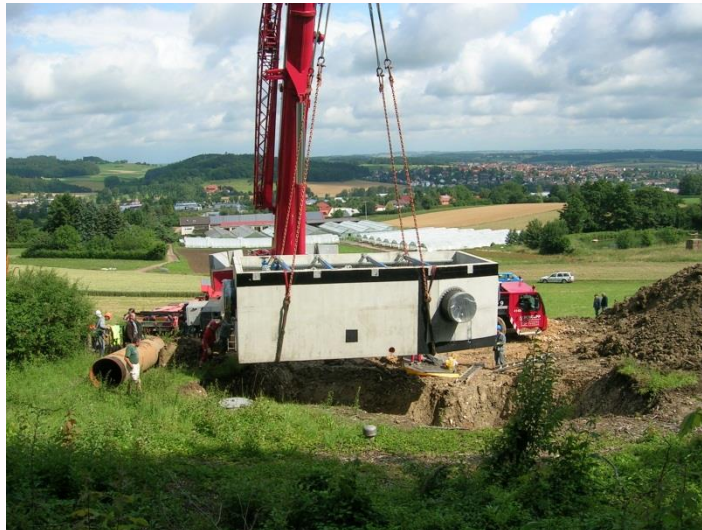
Fig. 23: Lifting the concrete cell with textile straps
