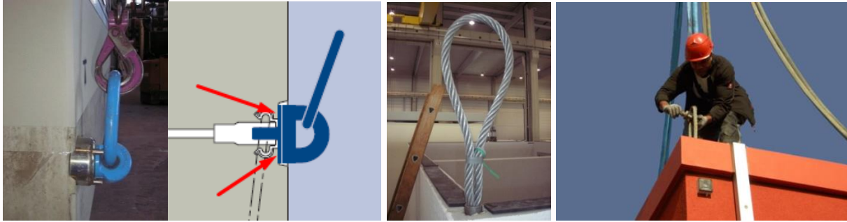
Fig. 21: Examples of correctly screwed lifting accessories
